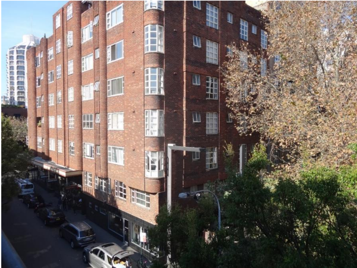
Figure 11: Neighbouring residential building at 113-115 Macleay Street, known as Gowrie Gate
