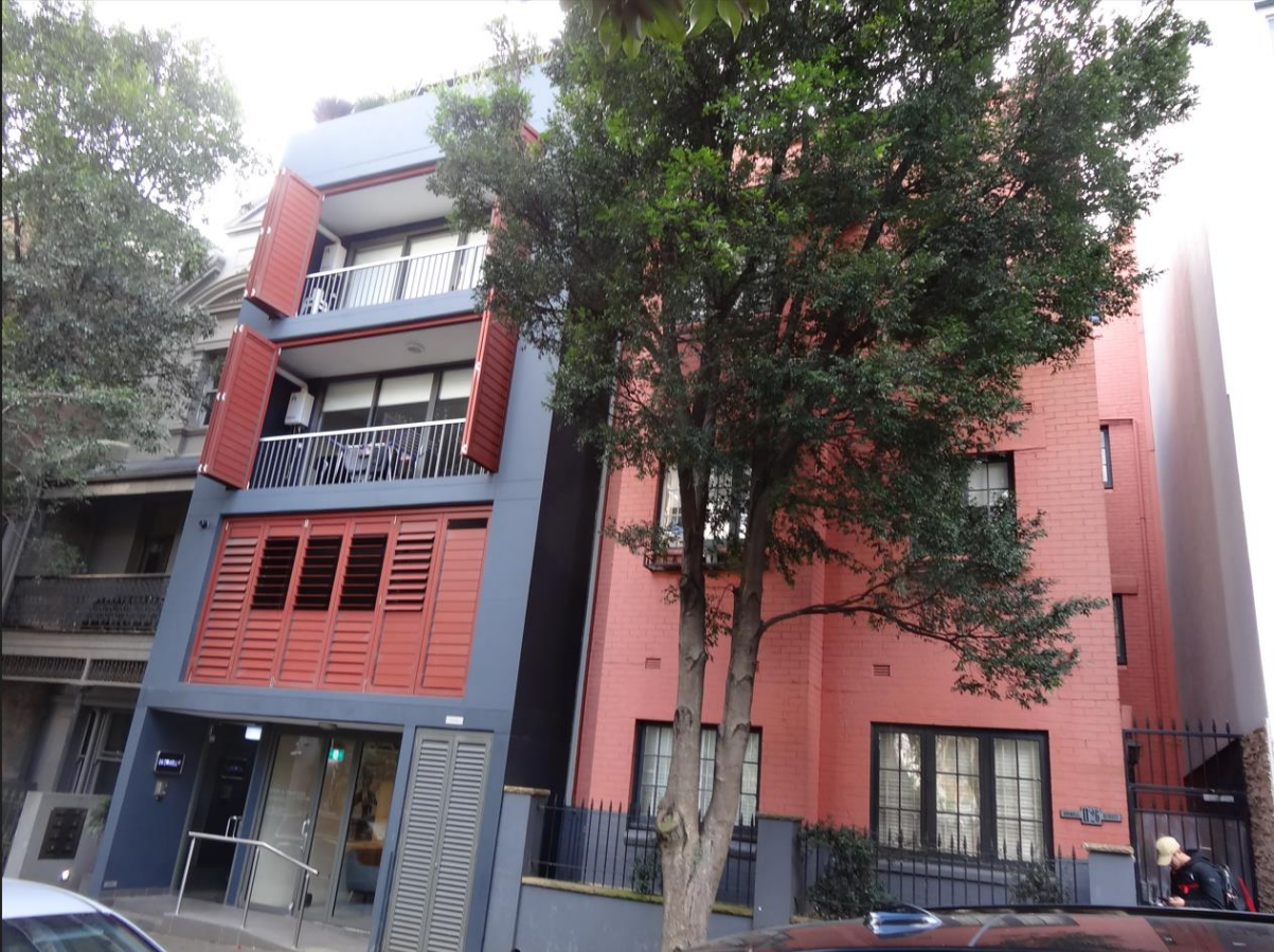
Figure 17: Neighbouring residential buildings at 24 and 26 Orwell Street
