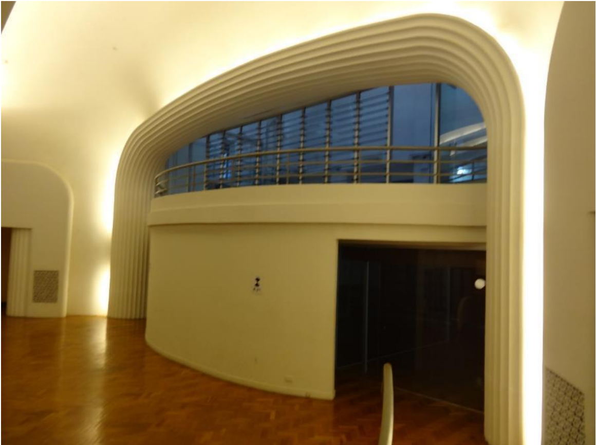
Figure 7: The existing stage and proscenium
