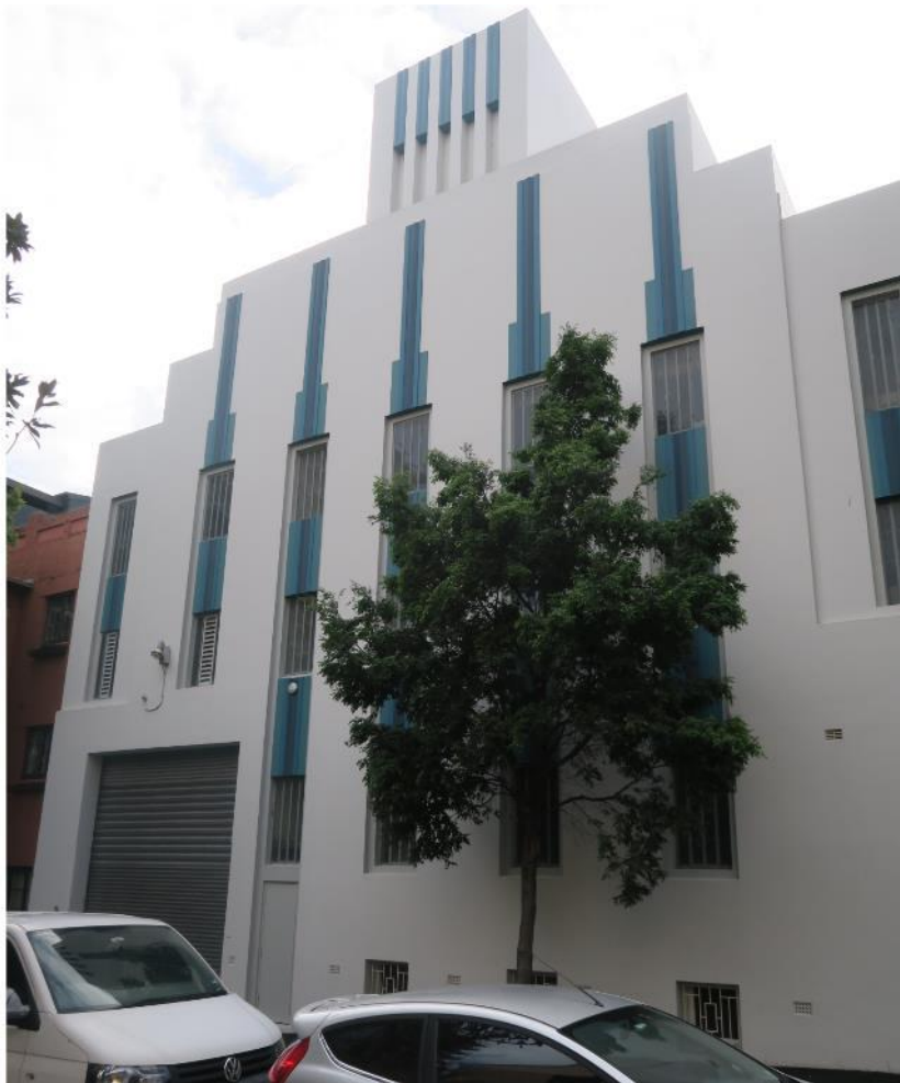
Figure 4: The flytower as viewed from Orwell Street, facing north
