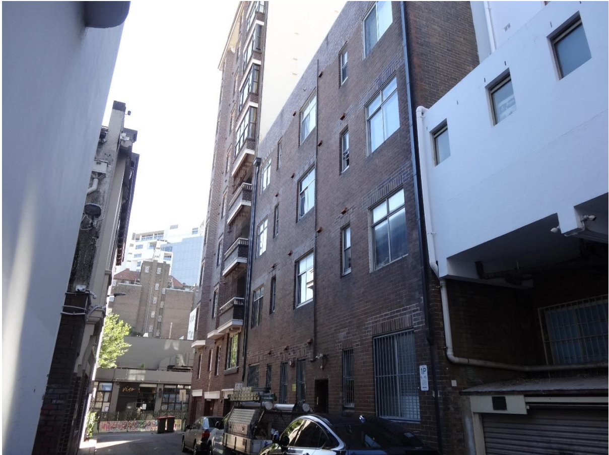
Figure 14: Neighbouring residential buildings on the opposite side of Orwell Lane looking north
